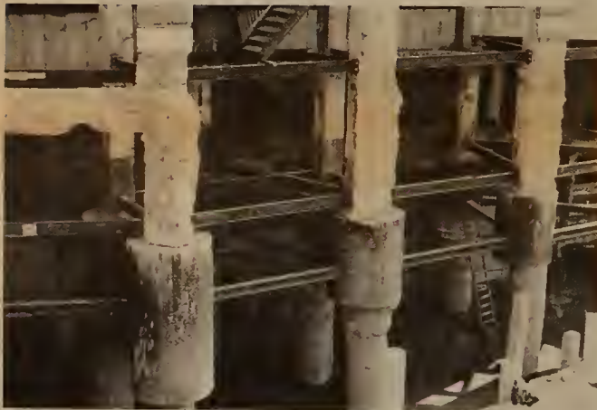
Underpinning of the Heath Building adjacent to Back Bay Station Site.
